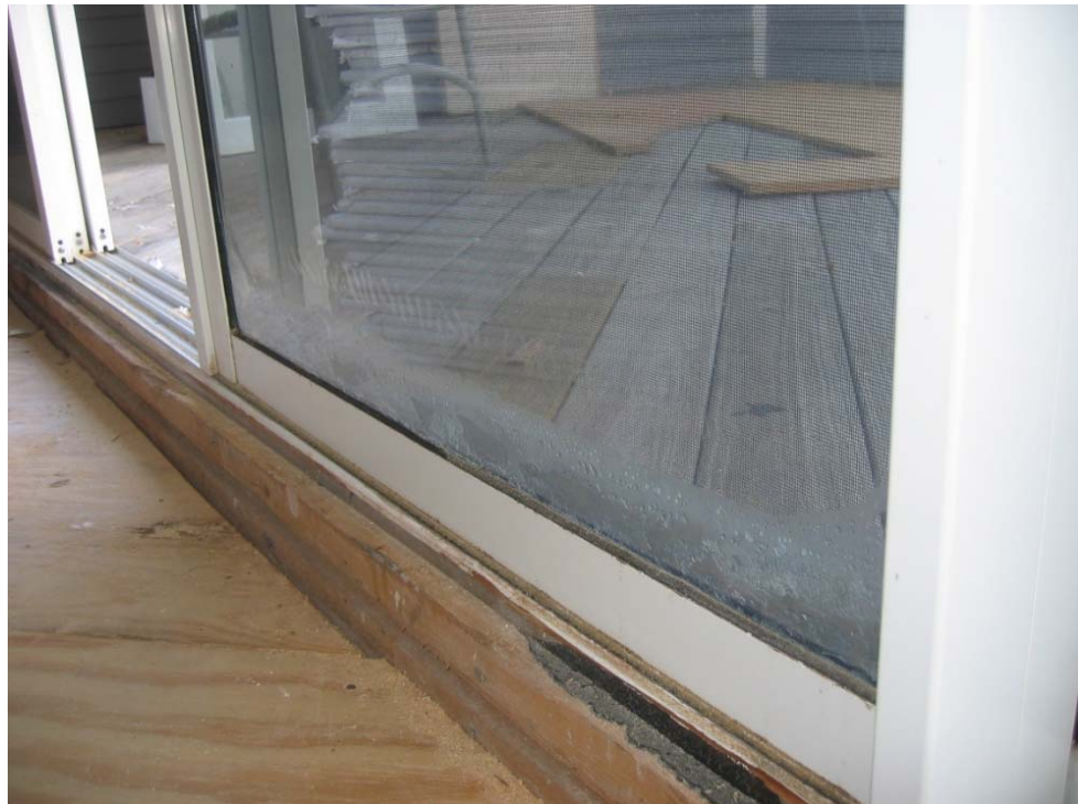
Figure 1: The widespread "Florida Glass Disease." Delamination of the PVB interlayer in an improperly designed framing.
