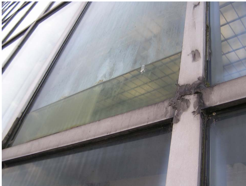
Figure 2: When all dams break loose, IGU may serve as an aquarium. The Metropolitan Museum of Art in New York City.
